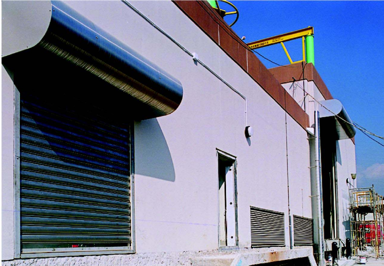
Stainless steel rectangular shape shutter hood with an access panel located in East Tsim Sha Tsui
