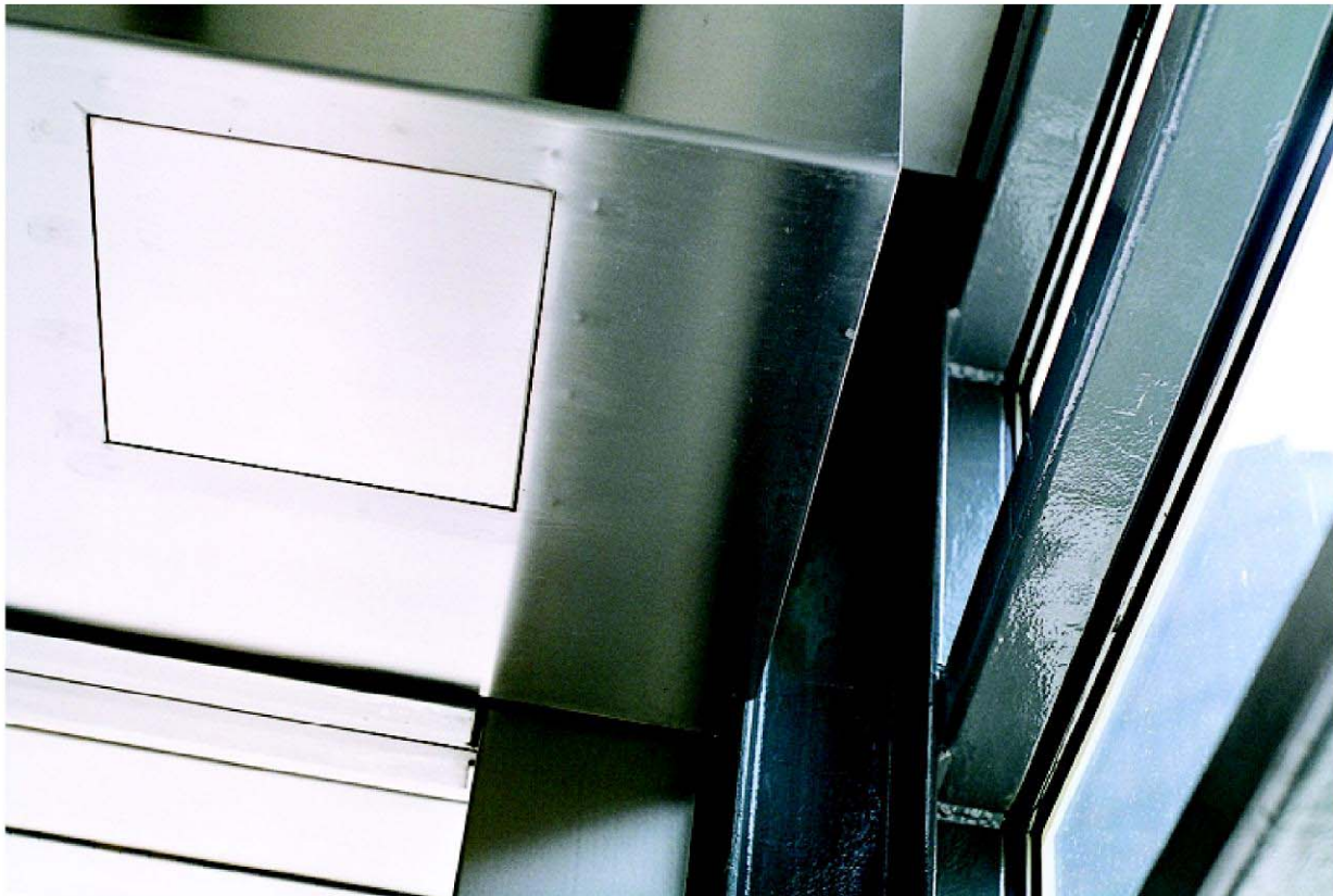
The access panel is for the maintenance inspection. Stainless steel rectangular shape shutter hood with an access panel located in East Tsim Sha Tsui station.
